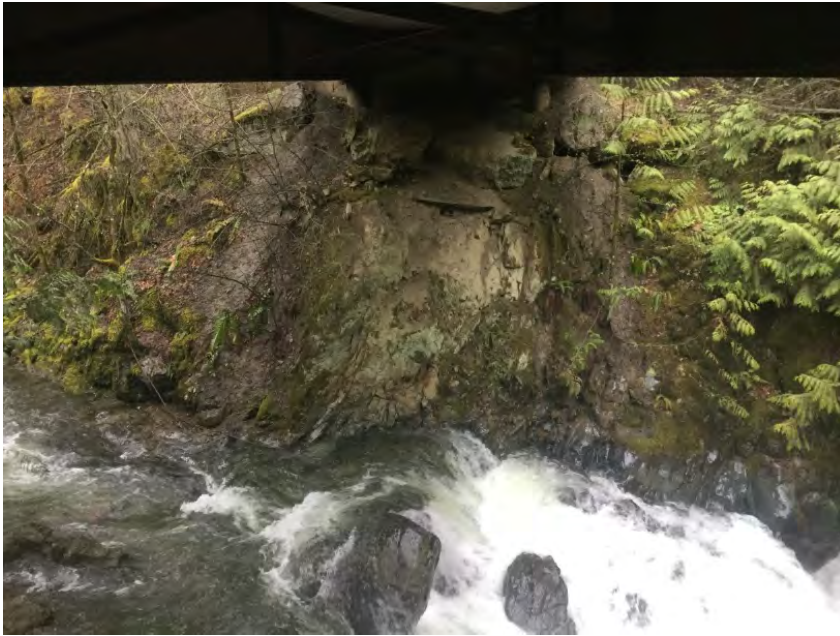
Left Bank Abutment when facing downstream
