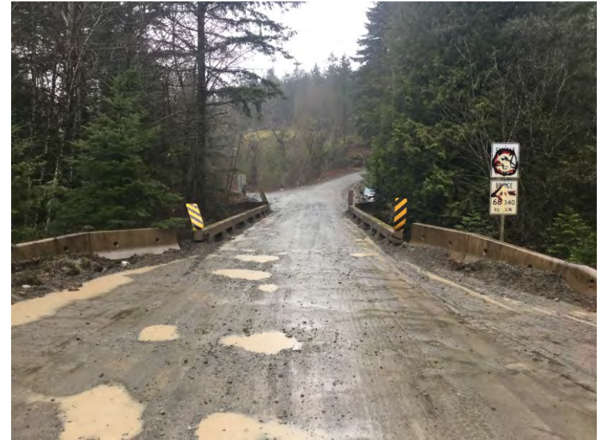
Approach from Right Bank when facing downstream
