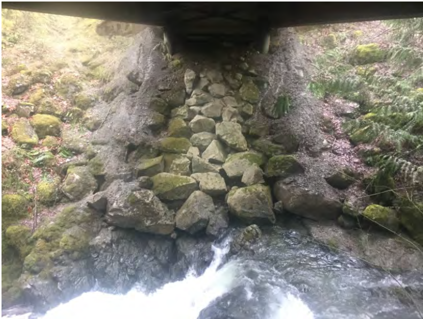
Right Bank Abutment when facing downstream
